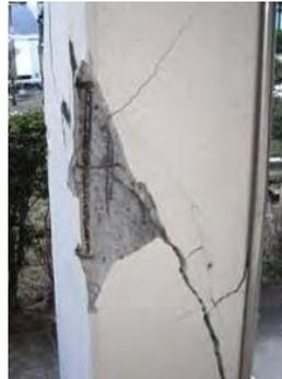
Figure 3.6. 1<sup>st</sup> storey shear cracks of column in Sendai [15].
