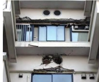
Figure 3.7. Damaged boundary beams with openings [15].
