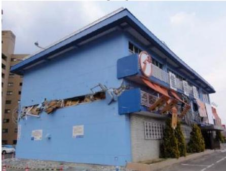
Figure 3.5. Collapse of a mid-story of a reinforced concrete building in Sendai [15].
